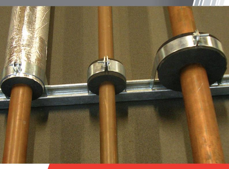
Thermobreak® Thermaloc is a lightweight and extremely tough closed cell polyethylene foam pipe support.
